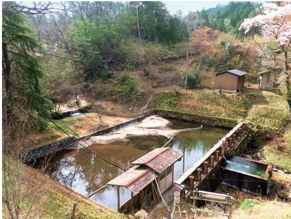
Photograph 4 Shirasaka flow-measuring weir
