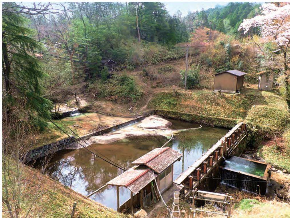
Photograph 4 Shirasaka flow-measuring weir
