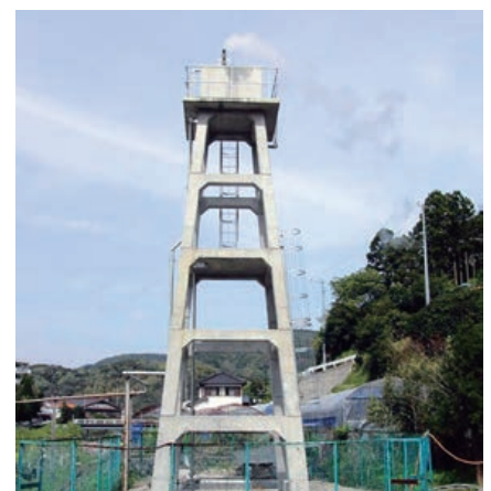
Photograph 2 Hot spring for heating of the greenhouse
