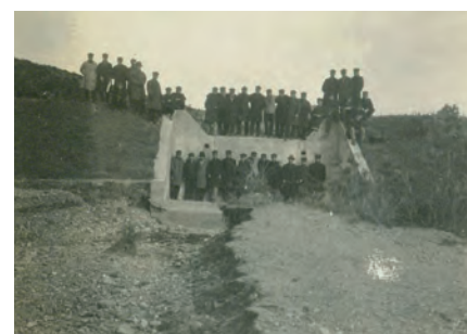
Photograph 7 Earth-fill weir with concrete drainage channel (photograph taken in 1929)
