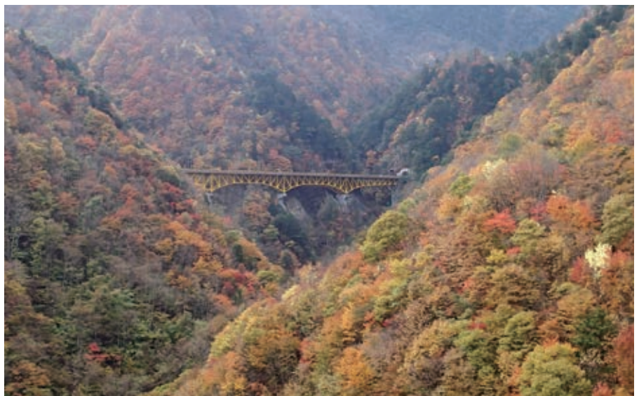
Photograph 2 V-shaped valley Mameyakizawa valley seen from the Mameyakibashi Bridge in front of the Karisaka Tunnel
