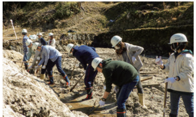
Photograph 3 Students removing sand from the weir
