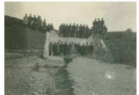
Photograph 7 Earth-fill weir with concrete drainage channel (photograph taken in 1929)
