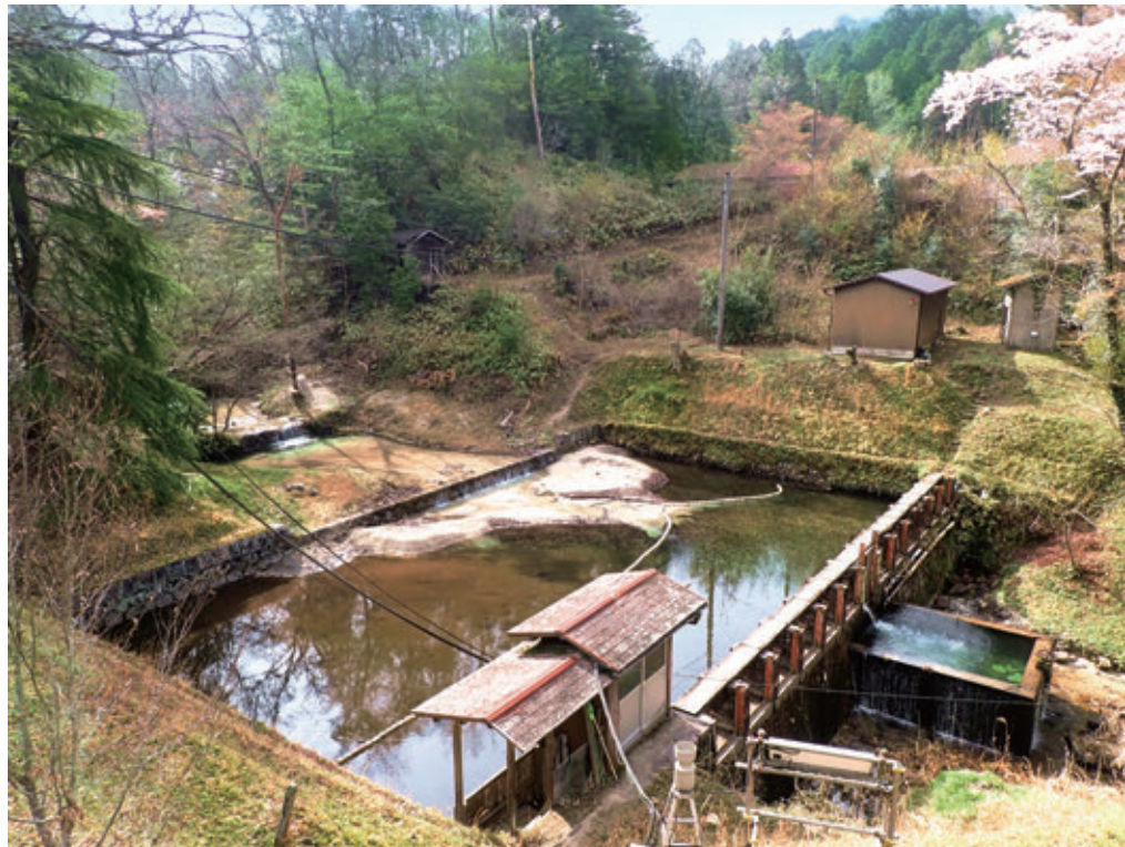
Photograph 4 Shirasaka flow-measuring weir
